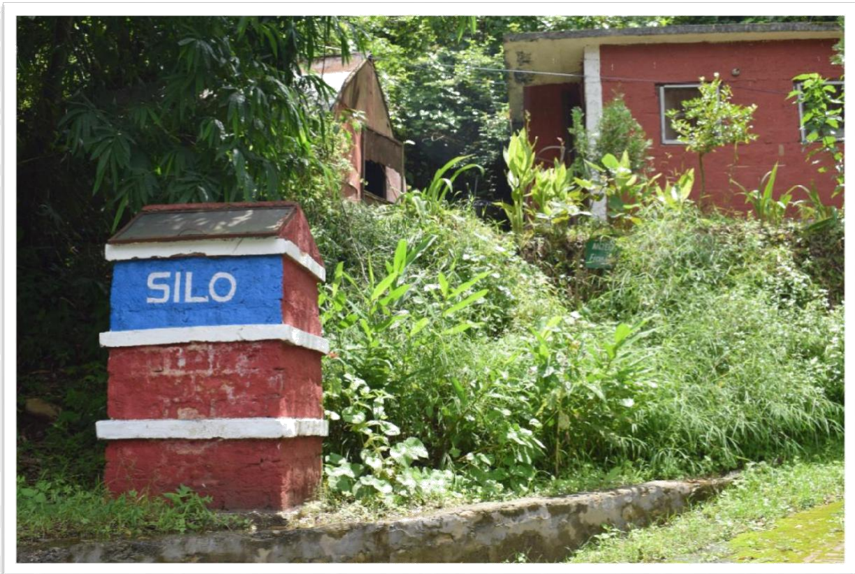
Image of a Degradabl Solid waste Bio- digester (SILO).
